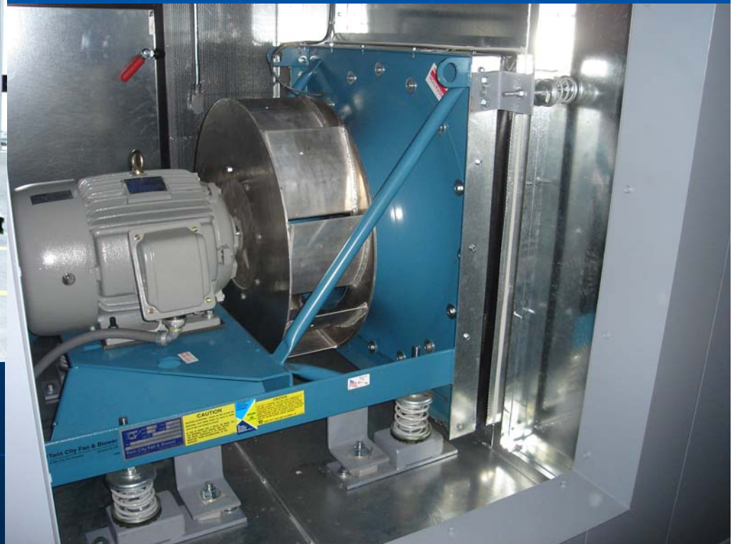
AMCA arrangement #4 "Direct Drive" Plenum Fan
